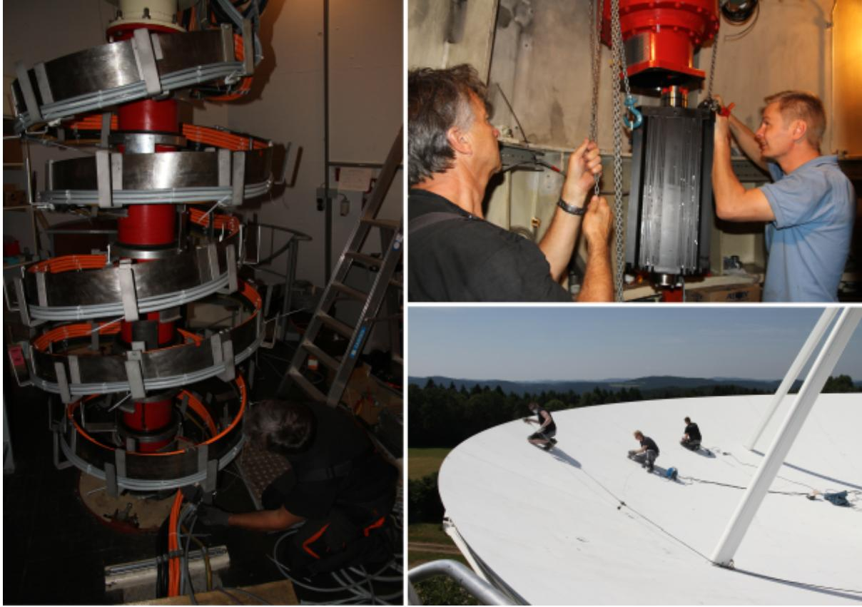
Figure 25: Wettzell RTW upgrade: **left** the new arrangement of the cable wrap with servo, power and coax cables **right top** finishing the gear drives and installing the new AC motors **right bottom** new coating and painting of the dish surface
