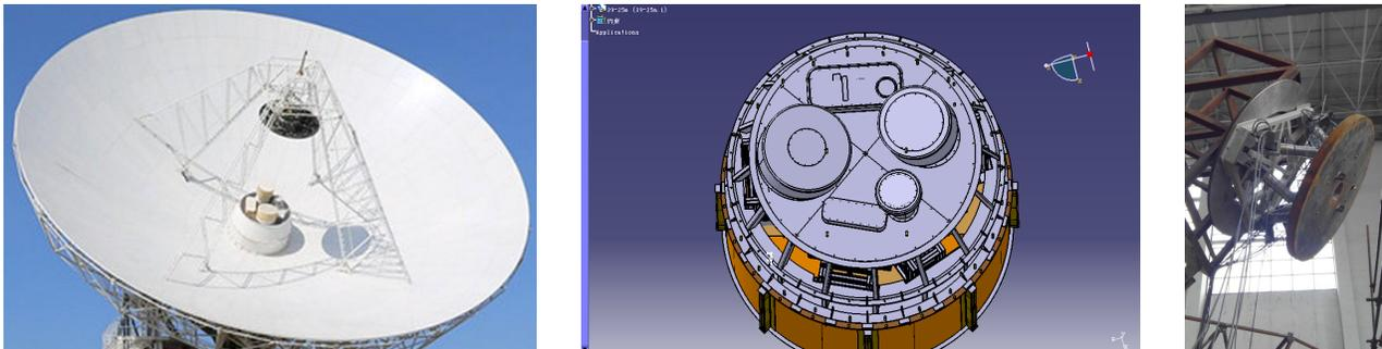
Figure 23: The new 26 m dish, new feed cabin design and secondary reflector Stewart platform
