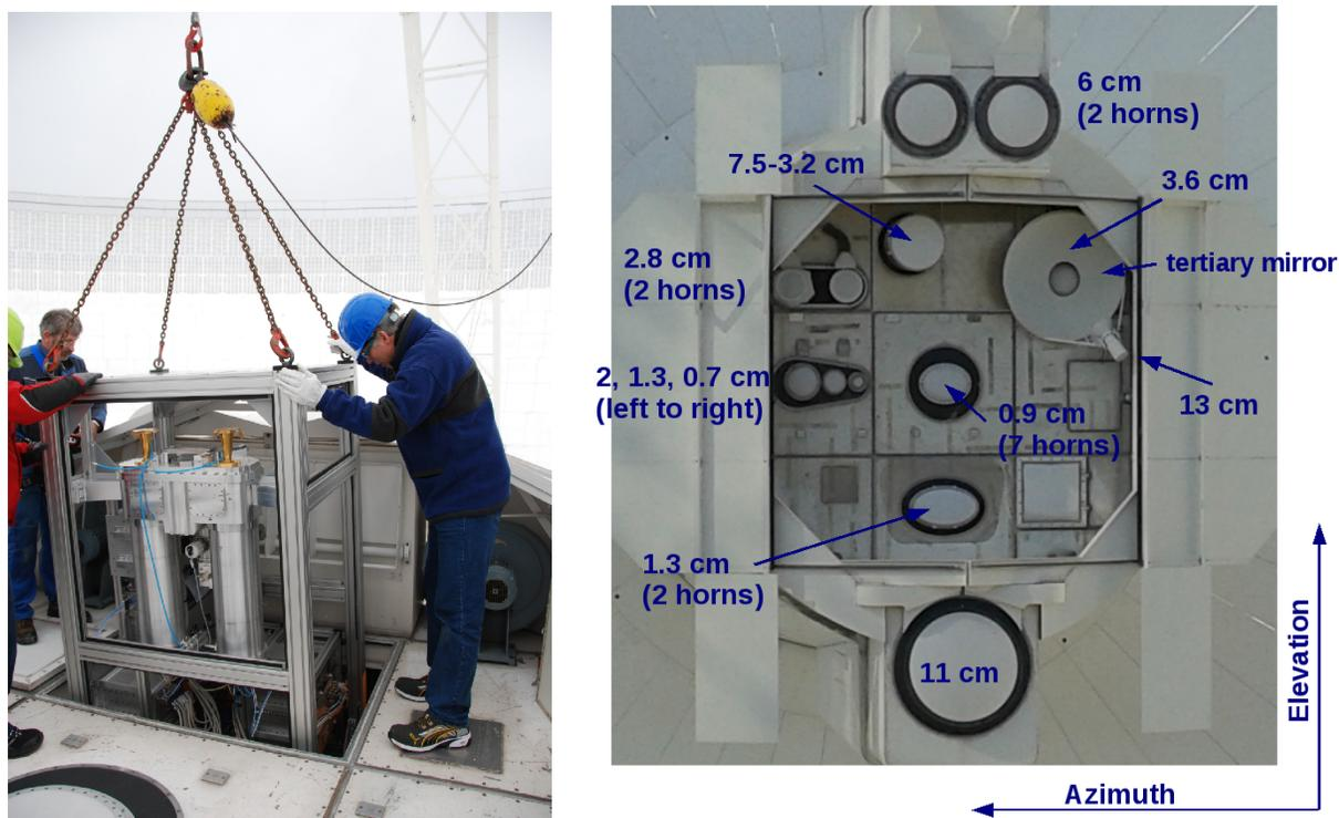
Figure 9: **Left:** Installing the new K-band receiver (photo: C.Kasemann) **Right:** Secondary focus feed arrangement
