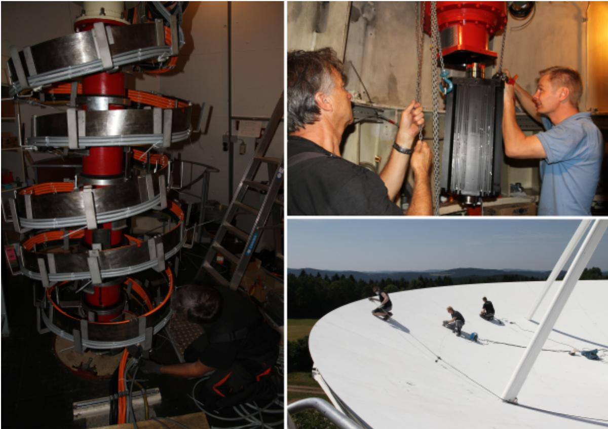
Figure 25: Wetzell RTW upgrade: **left** the new arrangement of the cable wrap with servo, power and coax cables **right top** finishing the gear drives and installing the new AC motors **right bottom** new coating and painting of the dish surface
