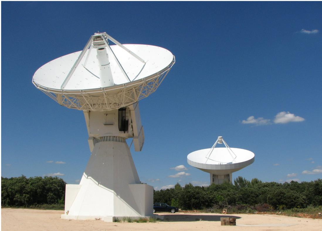
Figure 27: 13.2 m RAEGE radio telescope at Yebes, with 40 m telescope in background
