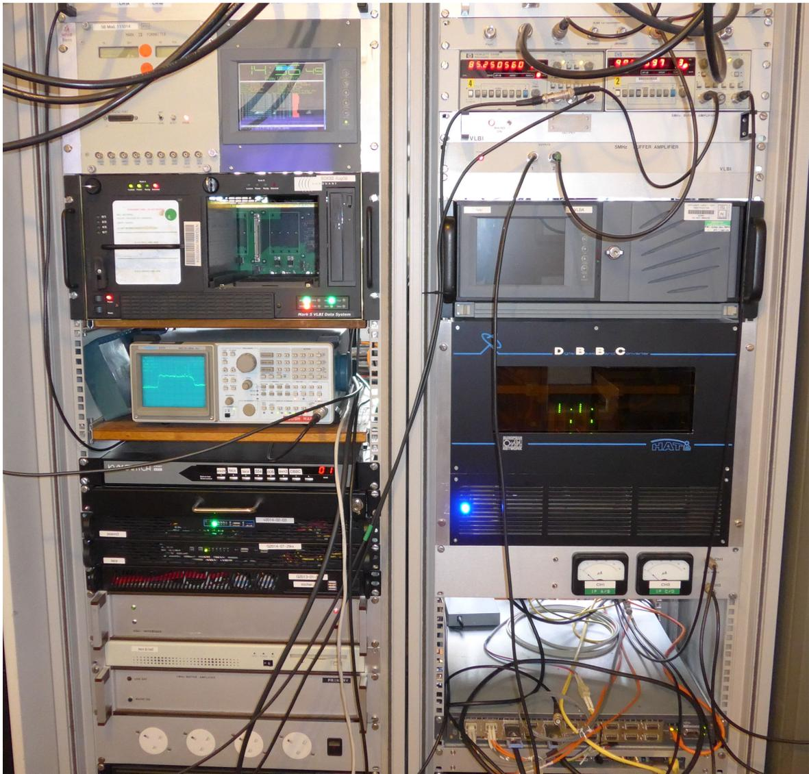
Figure 14: The VLBI racks including new DBBC unit
