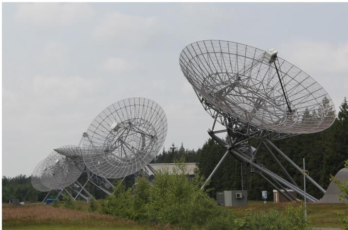
Figure 24: The image shows a partial view of the WSRT array, characteristic of the activities during 2014. The telescope in the foreground is part of the 3-dish array commissioning the prototype APERTIF frontends. The telescope in the middle is being refurbished, as part of the upgrade to APERTIF, while the other 3 telescopes (along with others, not seen here) are taking part in a VLBI observation.
