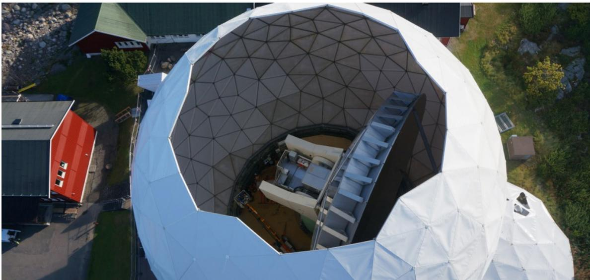
Figure 18: The top cap removed from the OSO 20m telescope radome.
